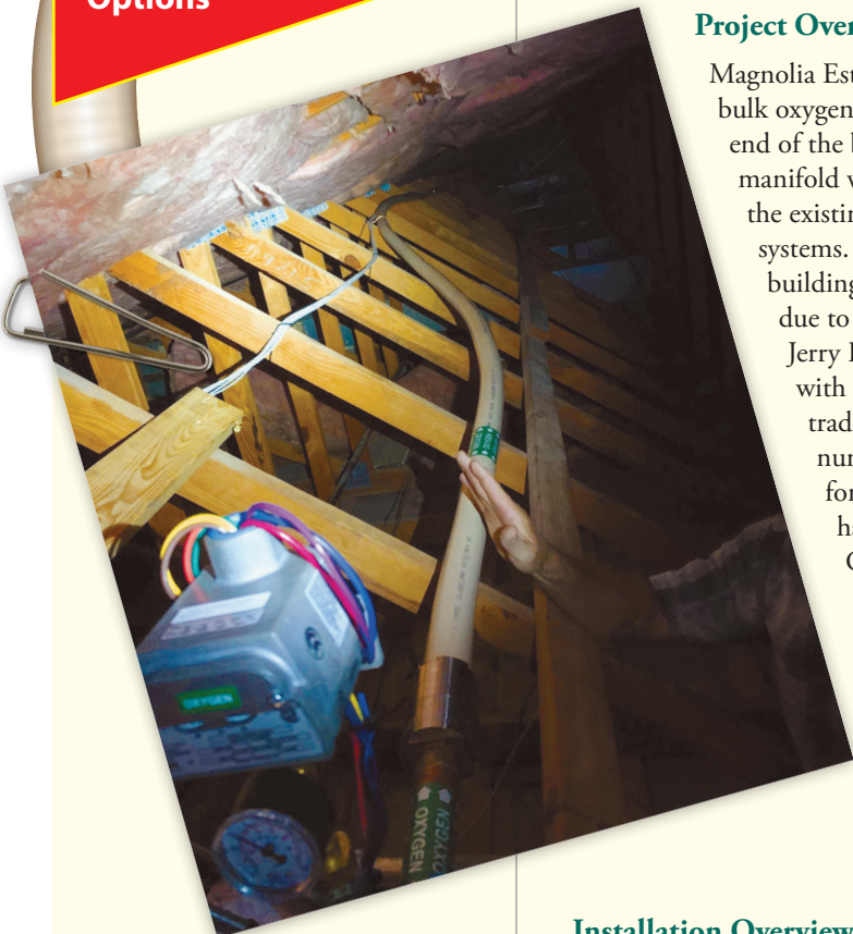
MediTrac® 1½" Tube and fitting connecting to oxygen new source valve line.
