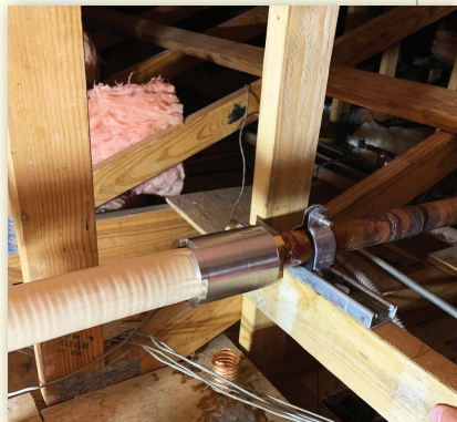
MediTrac® fitting tying into existing oxygen system.
