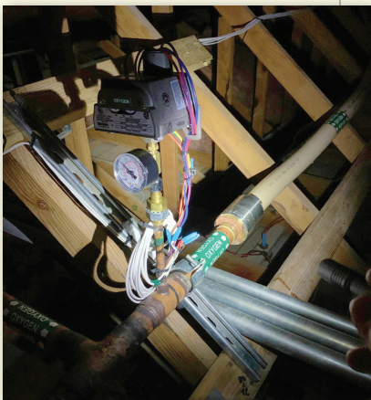
Completed 400' run of MediTrac ® under pressure test.
